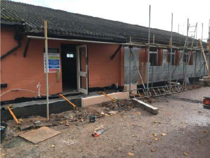
One of the first jobs - fixing the external insulation
