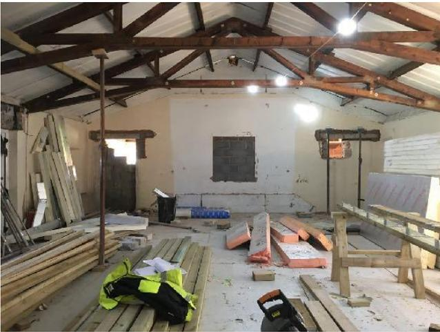
Work on installing the new roof started in the first week of the New Year and should be completed by the end of January. It's been decided to install 6 opening Velux roof lights instead of the proposed atrium. Two of these roof lights will be electrically operated. All will be fitted with blackout blinds.
